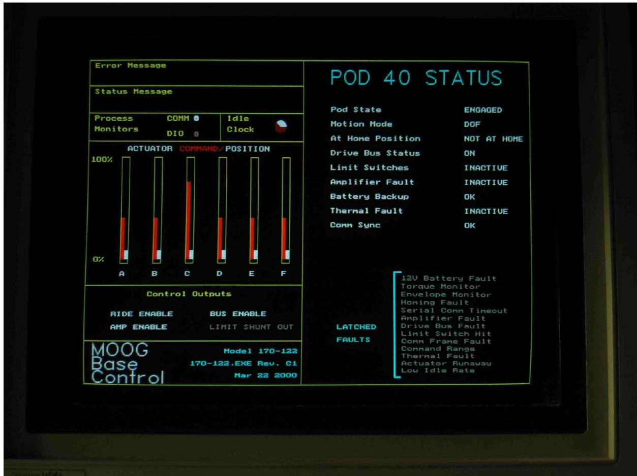
Figure 5. (c) The motion control system display in ENGAGED state,
